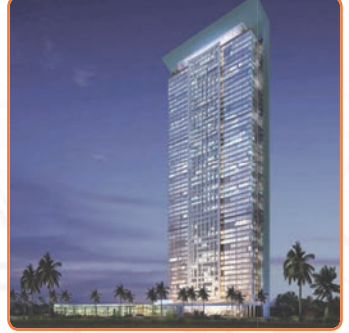
Al Rajhi Residential Tower
